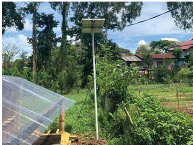
The very first solar panel in the district of Toraja, which is used to power an irrigation pump for an organic net zero vegetable garden.
