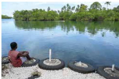
The islands’ locals protect their coasts from flooding with car tyres and cement.
