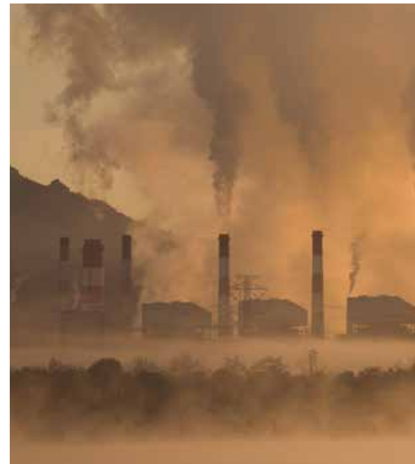
The Mae Moh coal power plant in Lampang, Thailand. Air pollution is a major burden of disease.
