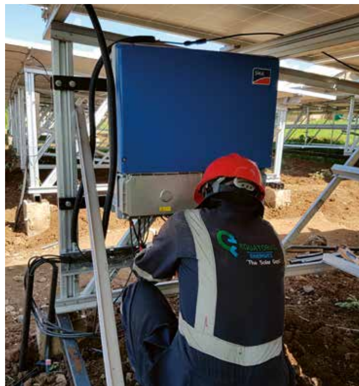
Solar PV technicians at work in Athi River, Kenya.
