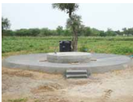
The catchment area of the rainwater harvesting pond is also utilised for drying and threshing crops.
